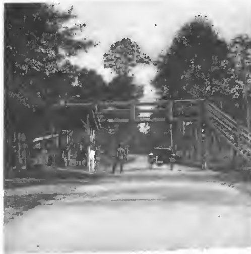
One of the Bridges Over the Course.
